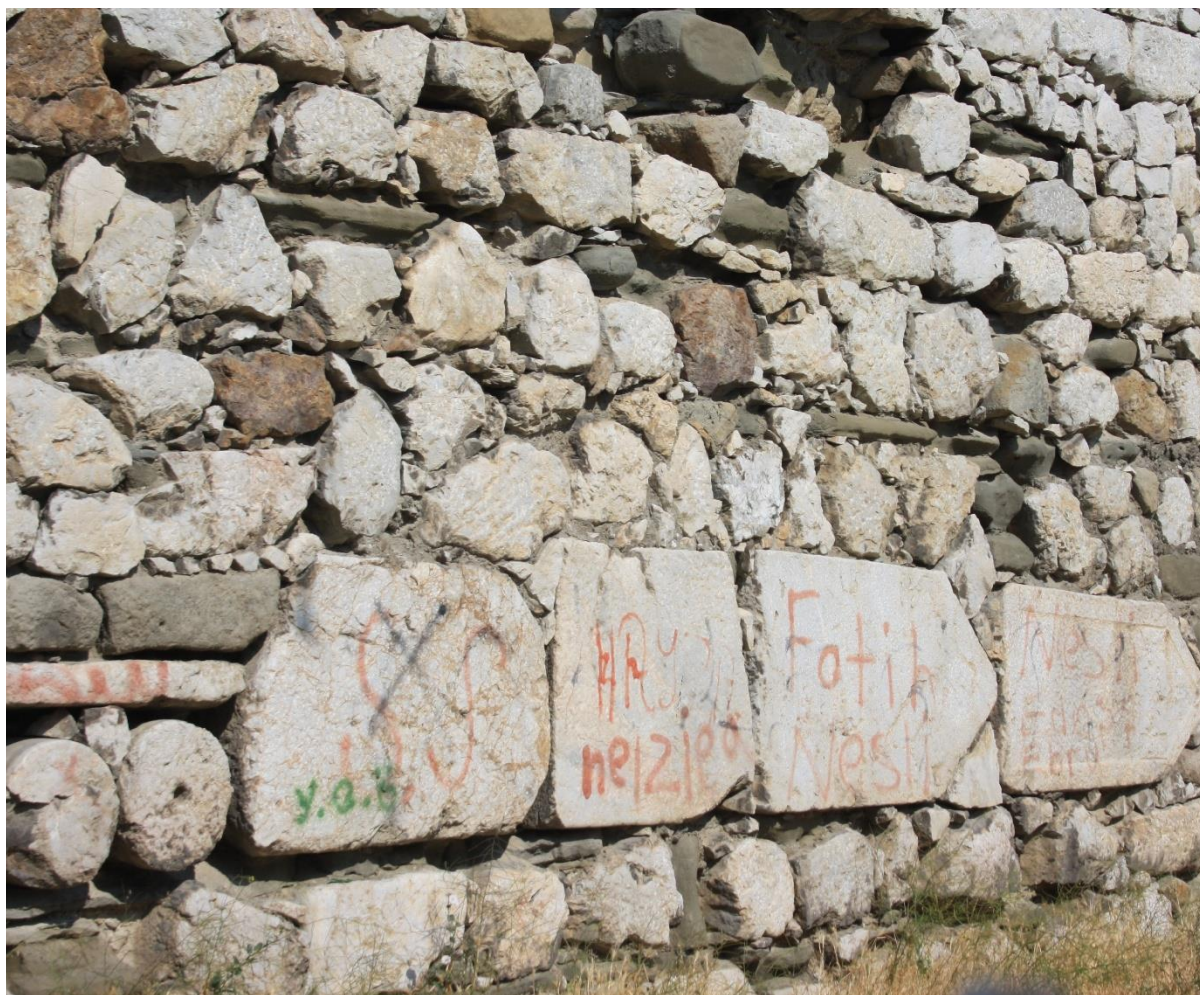
Fig. 8. Çorum: re-used ancient columns and grave steles in the stonework of the walls.
